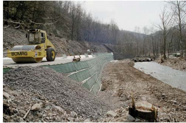
Figure 19. Geogrid reinforced railway embankment
