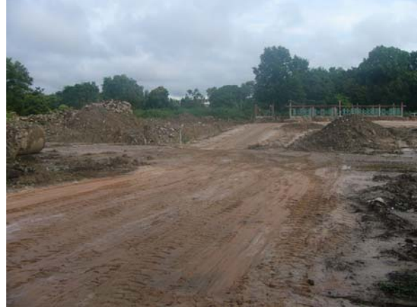
Figure 17. Limited rutting of reinforced base courses
