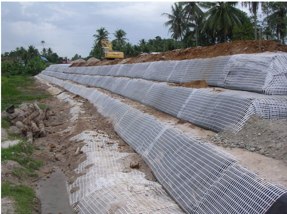
Figure 14. Reinforced slope during construction
