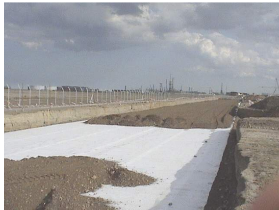
Figure 12. Installation of Secugrid® base course reinforcement
