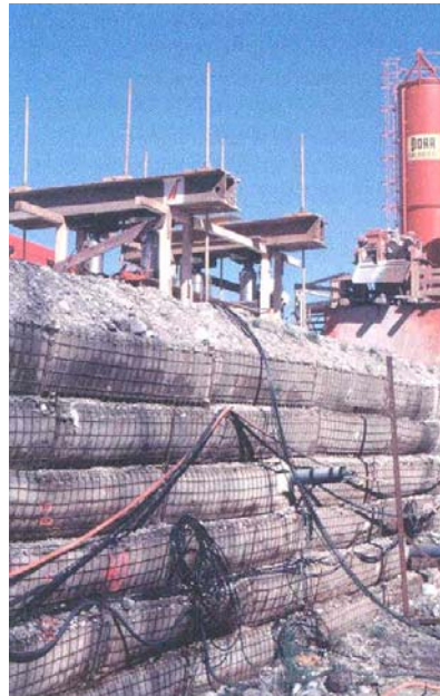
Figure 2. Testing the bearing capacity of a geogrid reinforced soil structure
