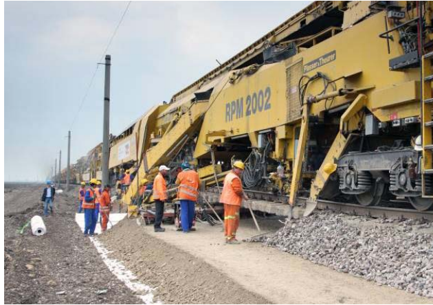
Figure 10. Installation of FPL & Ballast on Secutex® 251 GRK 4 and Secugrid® 30/30 Q1
